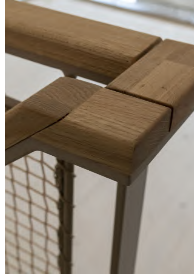
leuning hekwerk mezzanine in hout
